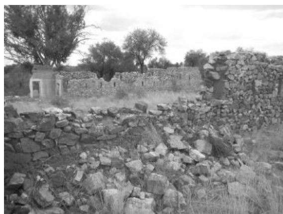
Photo 3. Partially collapsed walling QRS 350/3
