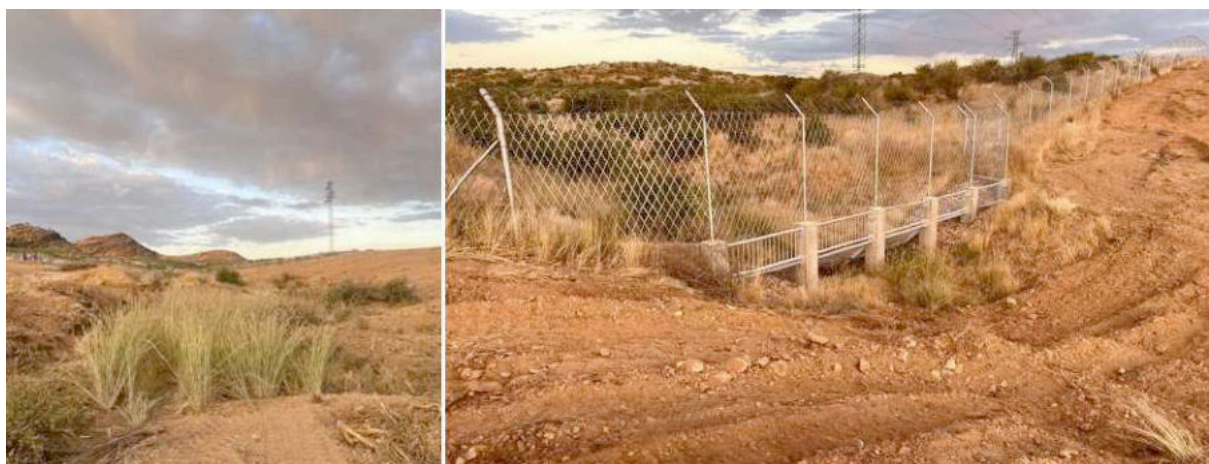
Figure 19: Drainage stream with tall grass and drainage sieving point
