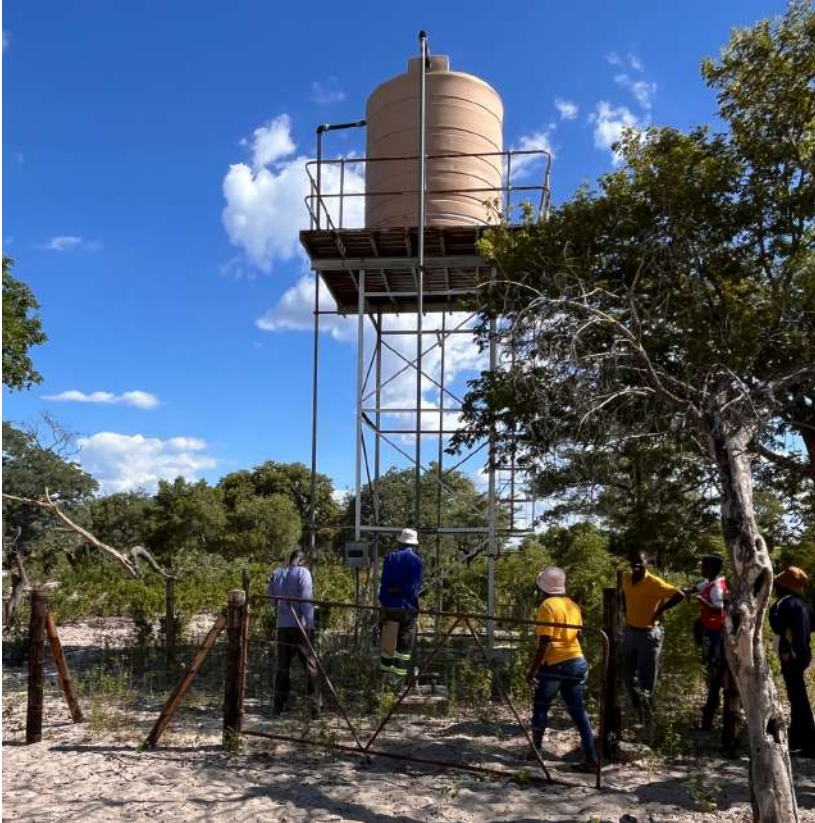
Figure 7. Broken borehole at Omundaungilo Settlement
