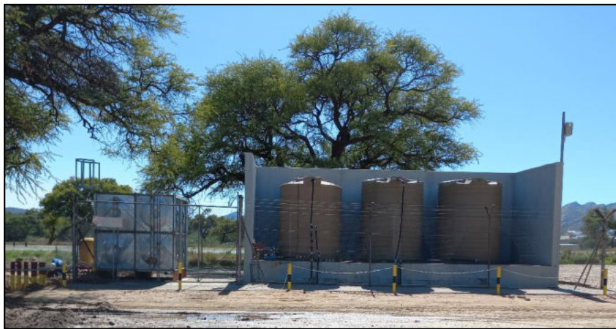
Figure 8: Water storage tanks
