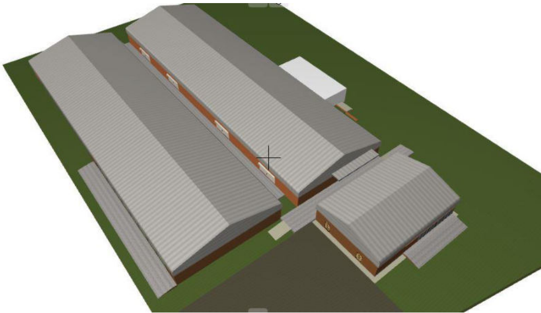
Figure 12: Aerial View of the Buildings
