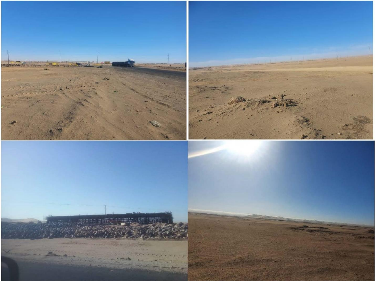
Figure 6: General area of the proposed development site, with road construction work on the interchange visible.
