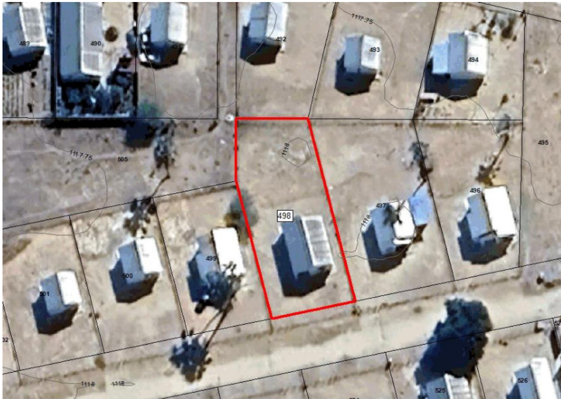
Figure 2: Aerial image of proposed project
