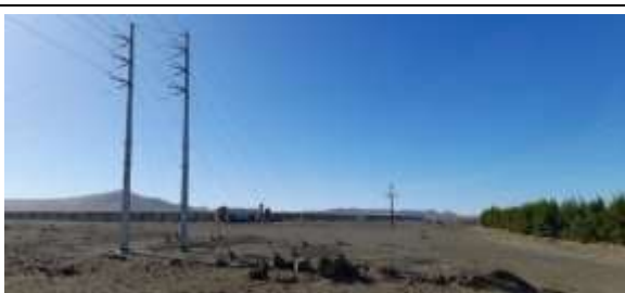
Photo 8-1 The existing solar plant and two existing power lines adjacent to the site
