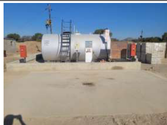
Photo 4-2 Spill slab at refuelling point
