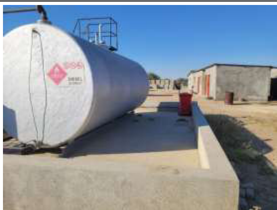
Photo 4-1 Existing storage tank inside a bund wall
