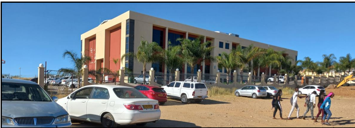
Figure 8: Lecture Hall next to the Erf (2)
