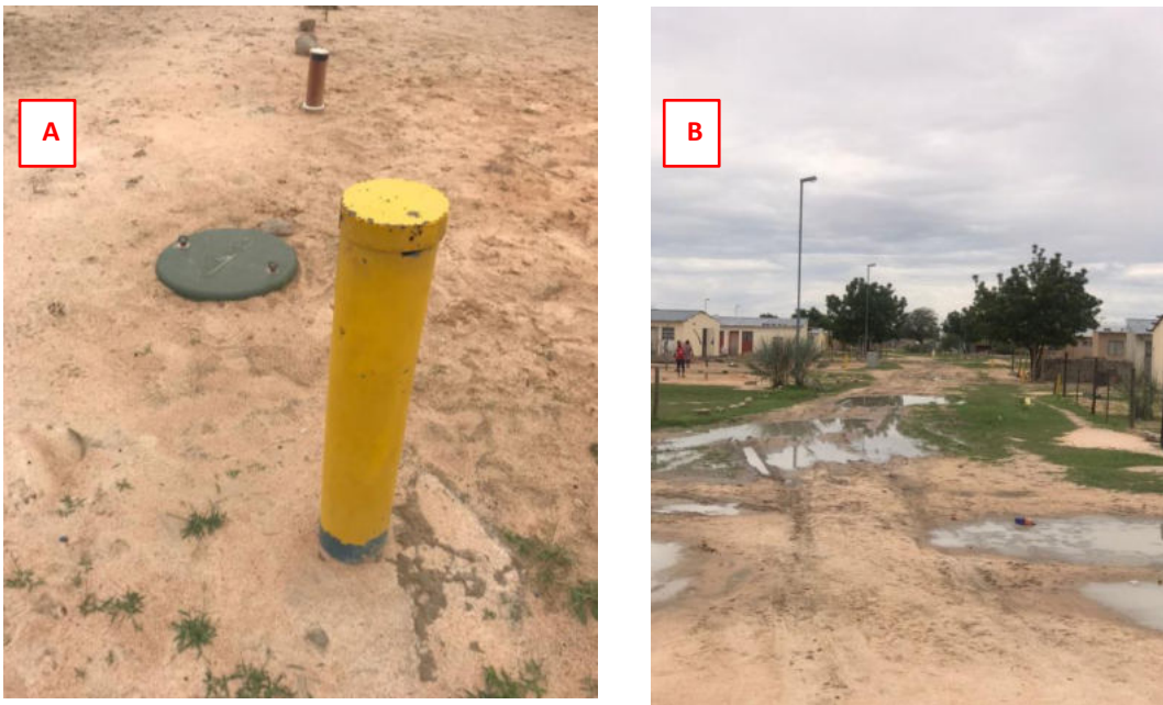
Figure 8: A – The vacuum sewer or pneumatic sewer system used and B - flooded streets in Erf 1499
