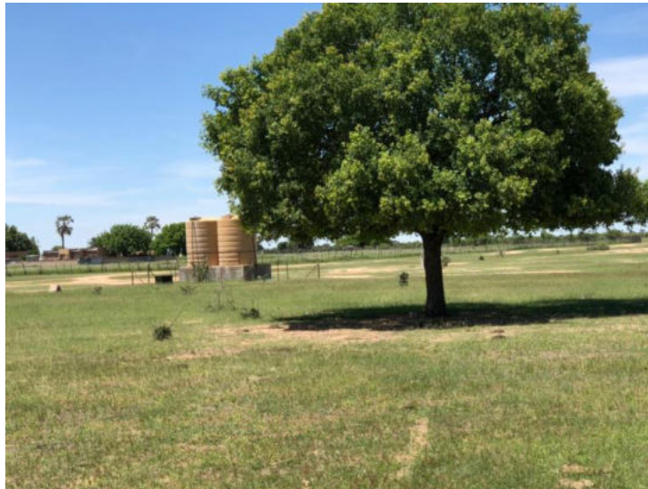
Figure 7: The communal water supply tanks on the Greenfield Portion
