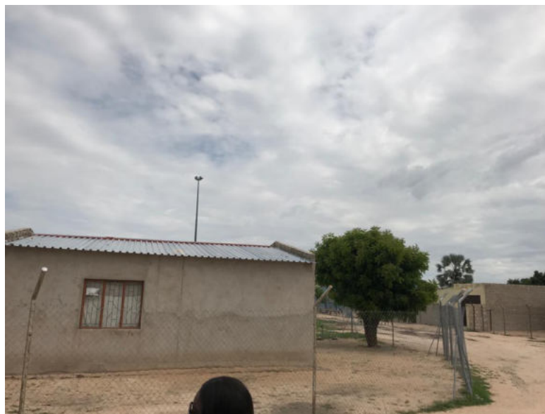
Figure 10: The type of housing on Portion 15
