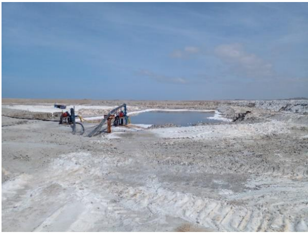
Wash water pond
