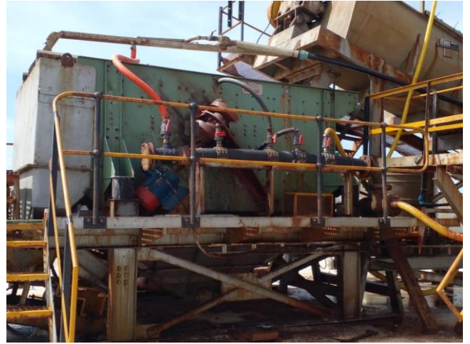
Serra wash plant
