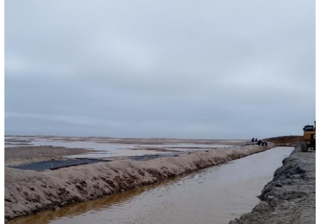
Wash water canal
