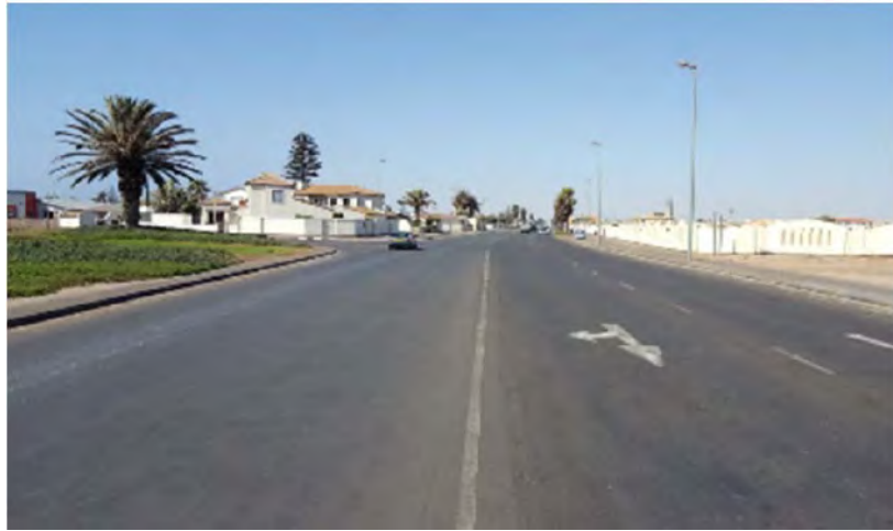
Photo 13: North-Eastbound View along Nangolo Mbumba at Esplanade Str
