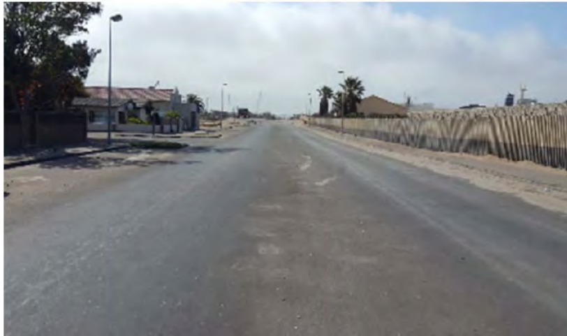
Photo 1: North-Westbound View along 5 th Road approaching KR Thomas Str
