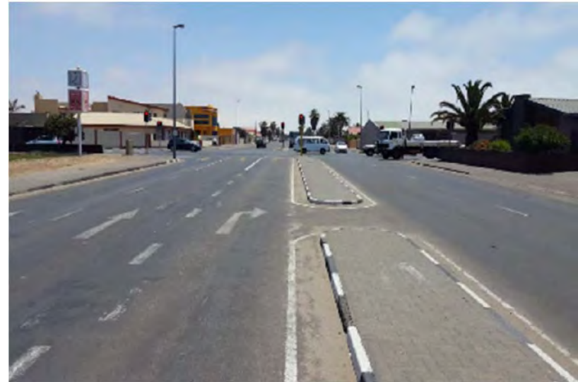
Photo 12: North-Westbound View along 5 th Road at Nangolo Mbumba
