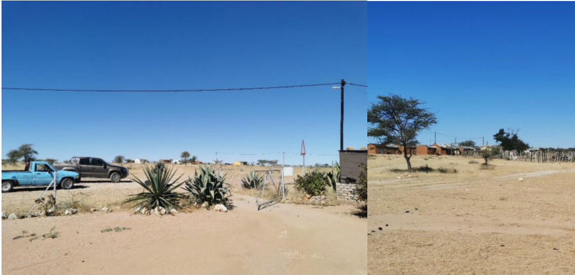
Figure 24: The powerline supplying the Okamapuku Village
