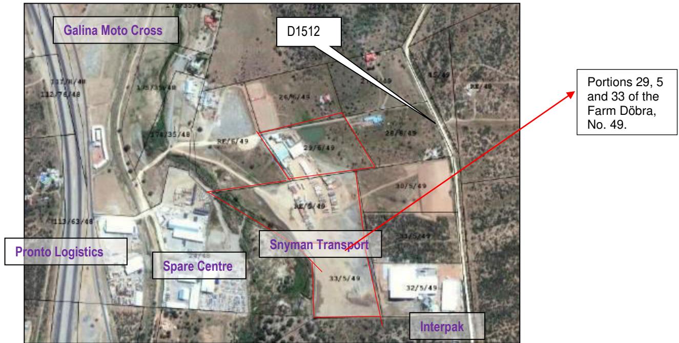
Figure 11: Image showing the activities around the portions
