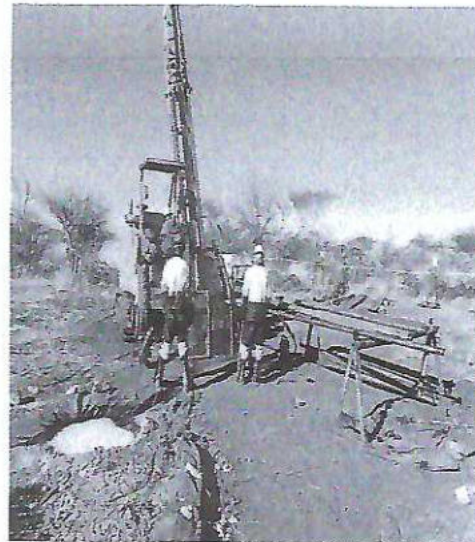
Drill-rig and sumps
