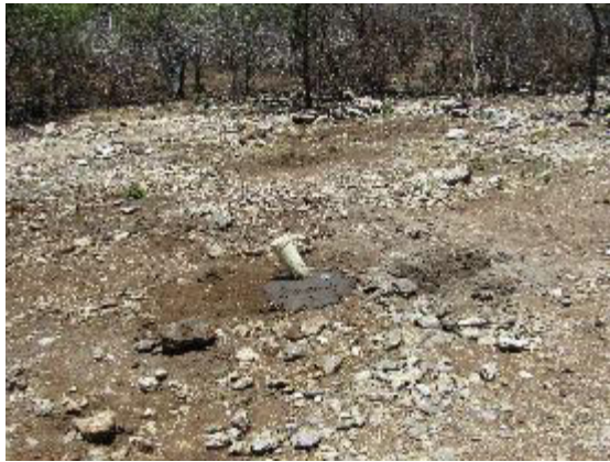
Post drilling - cleaned drill-site & capped hole
