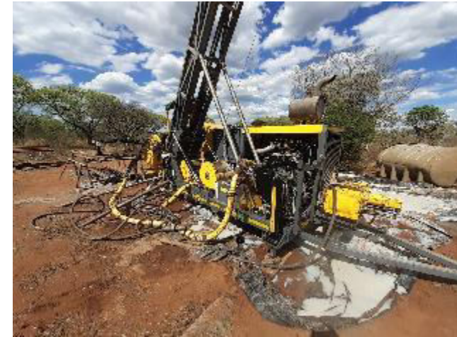
Drill rig and sumps
