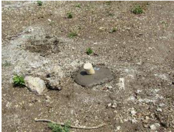
Post drilling - cleaned drill-site & hole capped
