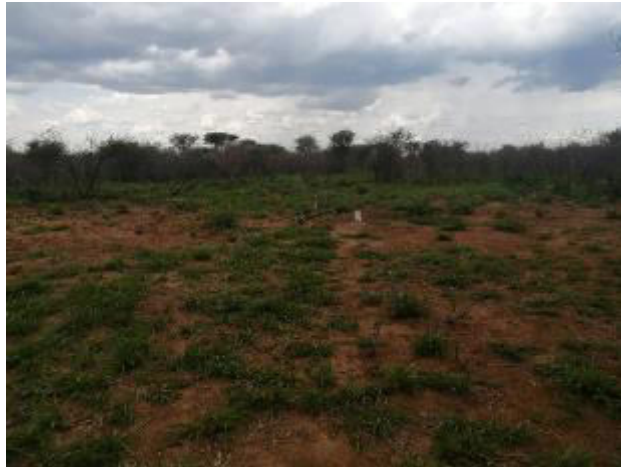
Post drilling - cleaned drill-site & hole capped
