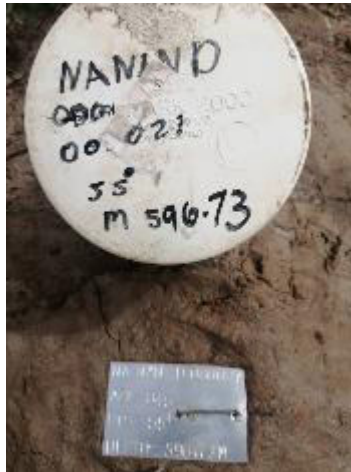
Post drilling - cleaned drill-site & capped hole
