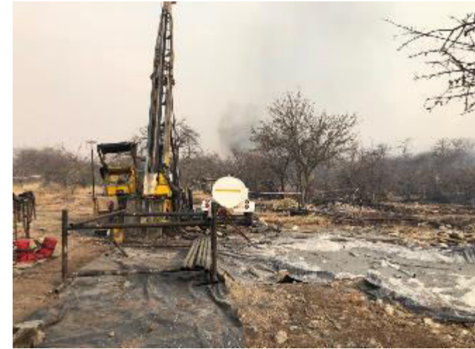
Drill rig and sumps
