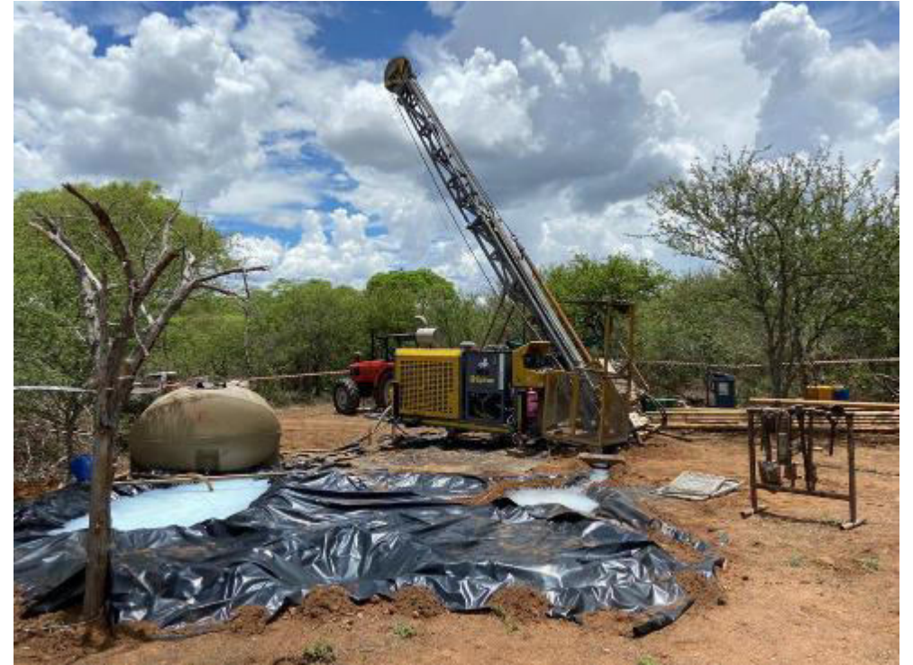
Drill rig and sumps
