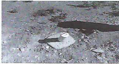
Post drilling - cleaned drill-site & hole capped
