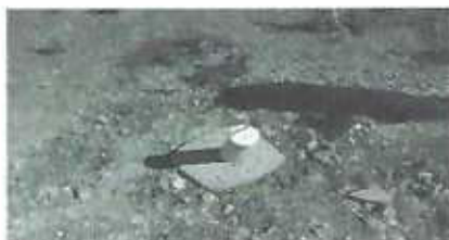
Post drilling - cleaned drill-site & hole capped
