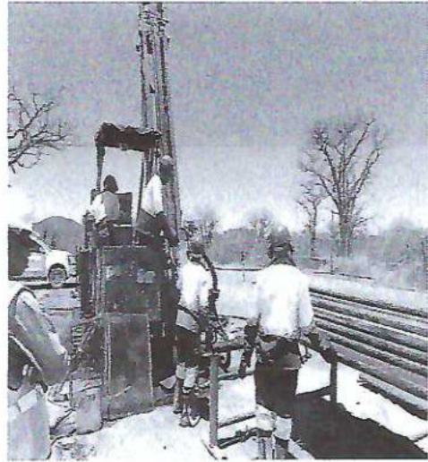
Drill rig and sumps
