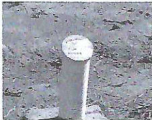
Post drilling - cleaned drill-site & capped hole
