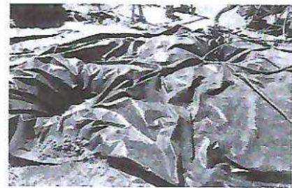
Plastic liner - preparing sump
