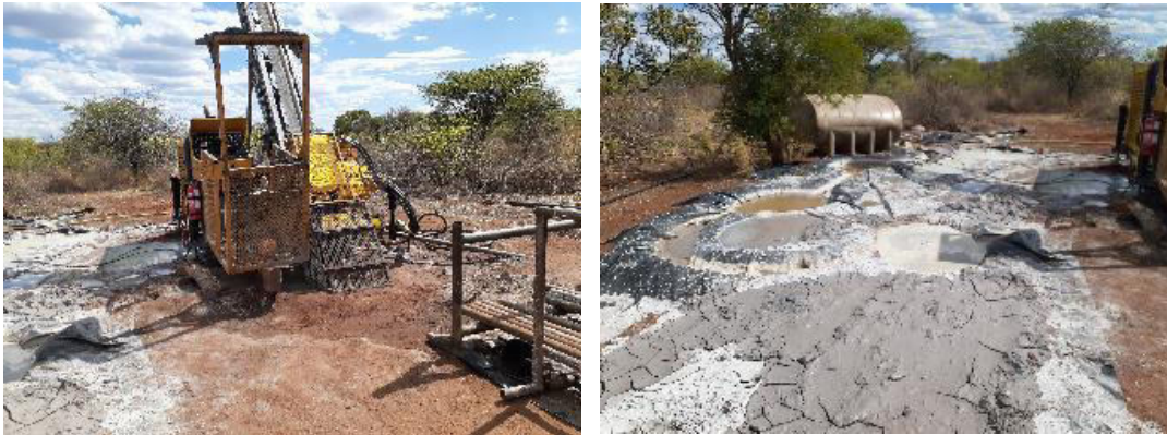
Figure 26 - Drill rig and sumps at site: NANAND000026
