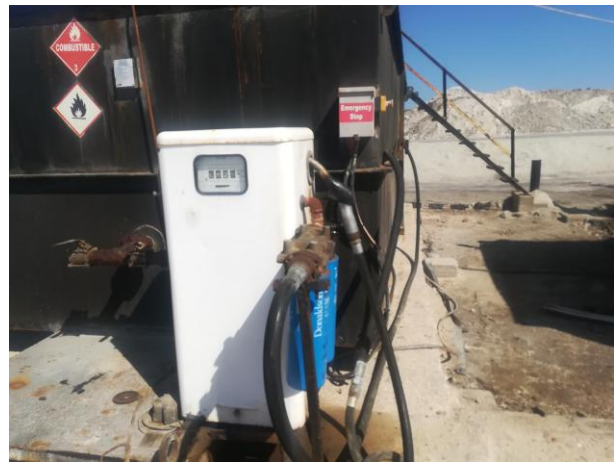
Photo 2. Dispenser on concrete containment floor
