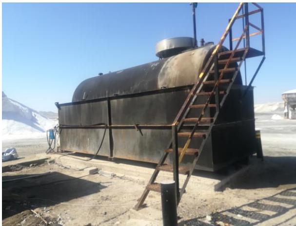
Photo 1. Existing 23m 3 tank in containment structure
