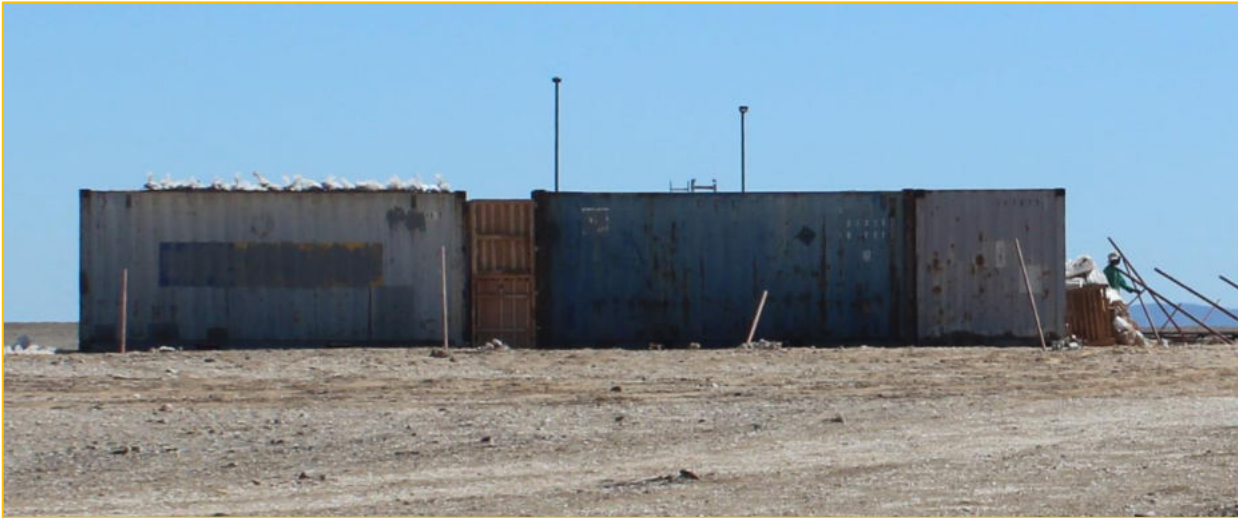
Figure 6: Shows current status of the Base-camp facility consisting of old shipping containers left by previous license holder
