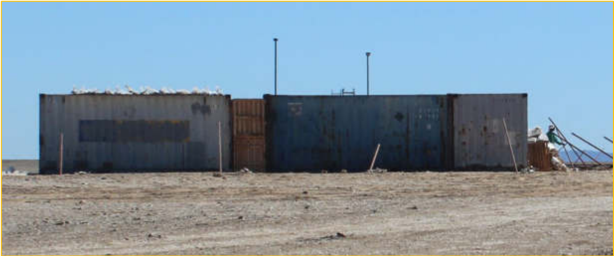
Figure 4: Shows current status of the Base-camp facility consisting of old shipping containers left by previous license holder
