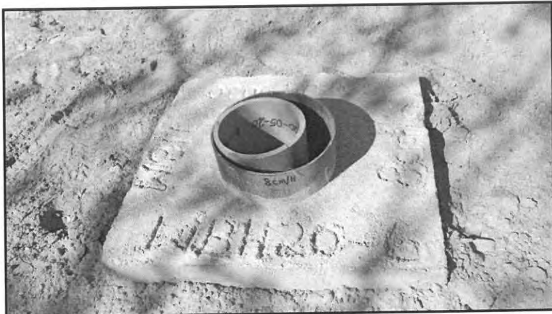
Plate 4: One of the two recently drilled water boreholes.
