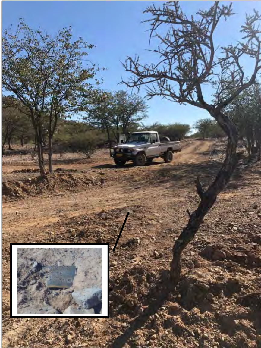
Plate 3: Rehabilitated Diamond Drill site. The borehole is covered with a steel plate (insert) and sumps are refilled and the area is raked. Mopane (in the background) and Witgat (in the foreground) trees are not harmed during exploration activities.
