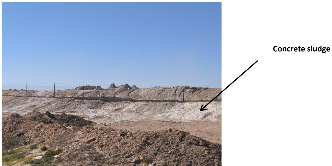
Figure 5: Concrete sludge flowing from the dumpsite into the surrounding environment
