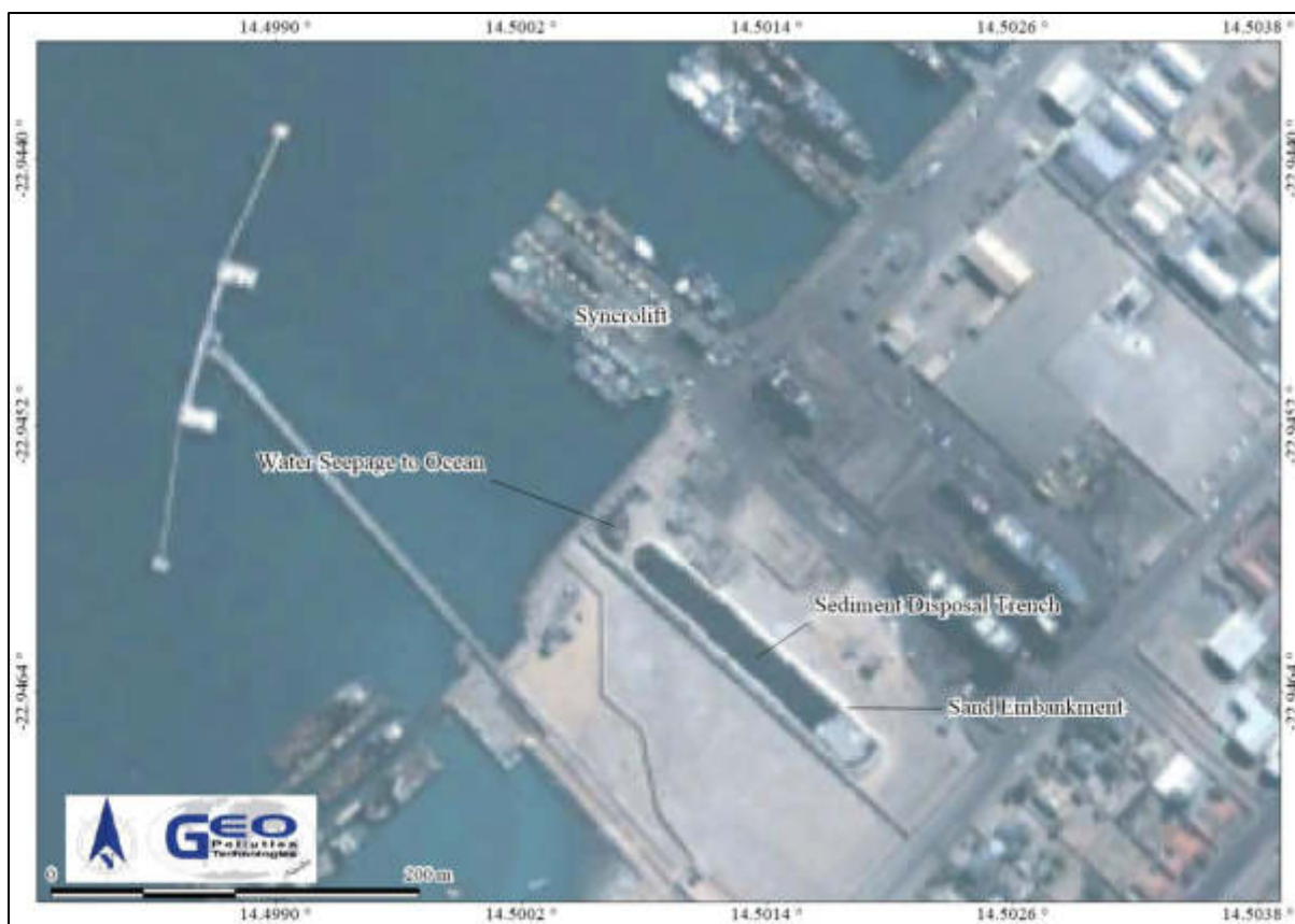
Figure 6-4 Onshore disposal site (Google Earth 06/2007)
