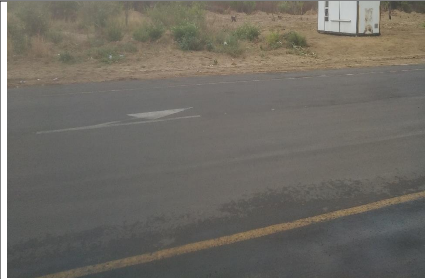
View of Wenela main road that provides access to the site
