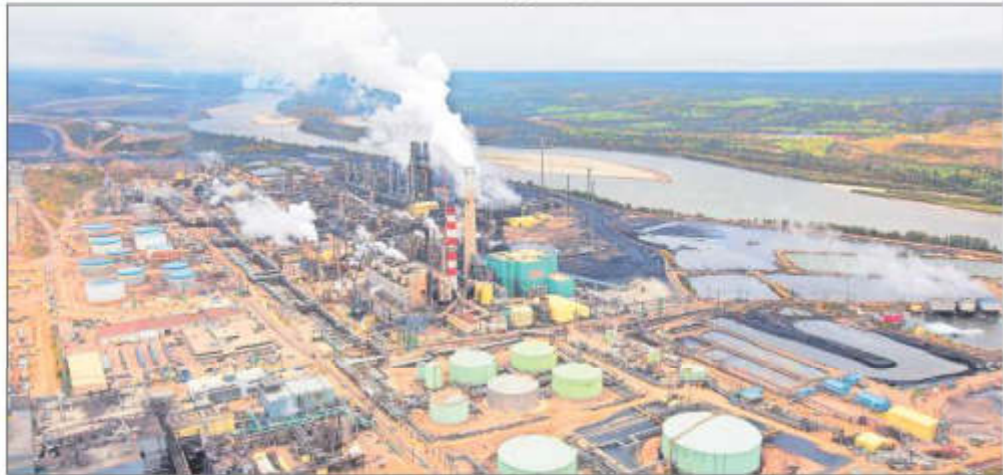
The Suncor oil sands processing plant near the Athabasca River at their mining operations near Fort McMurray, Alberta, September 17, 2014. REUTERS/TODD KRODL/FILE PHOTO
