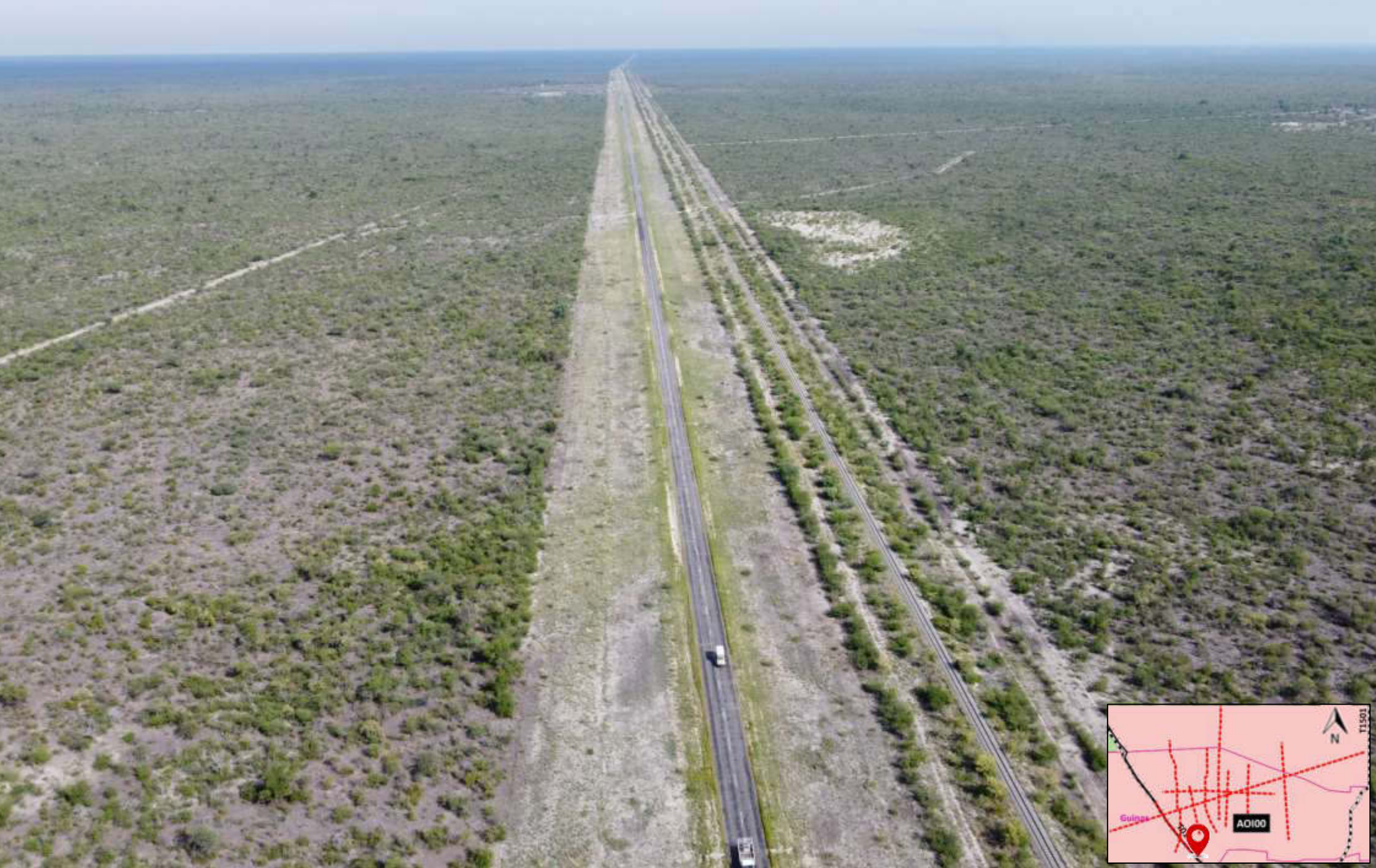
Plate 1.30: Southern section of Line 11, running along the B1 Road from Tsumeb to Oshivelo, drone image view to the north. MEL 2D Seismic Survey Operations - 40 - EMP Report for PEL 93-APR 2022
