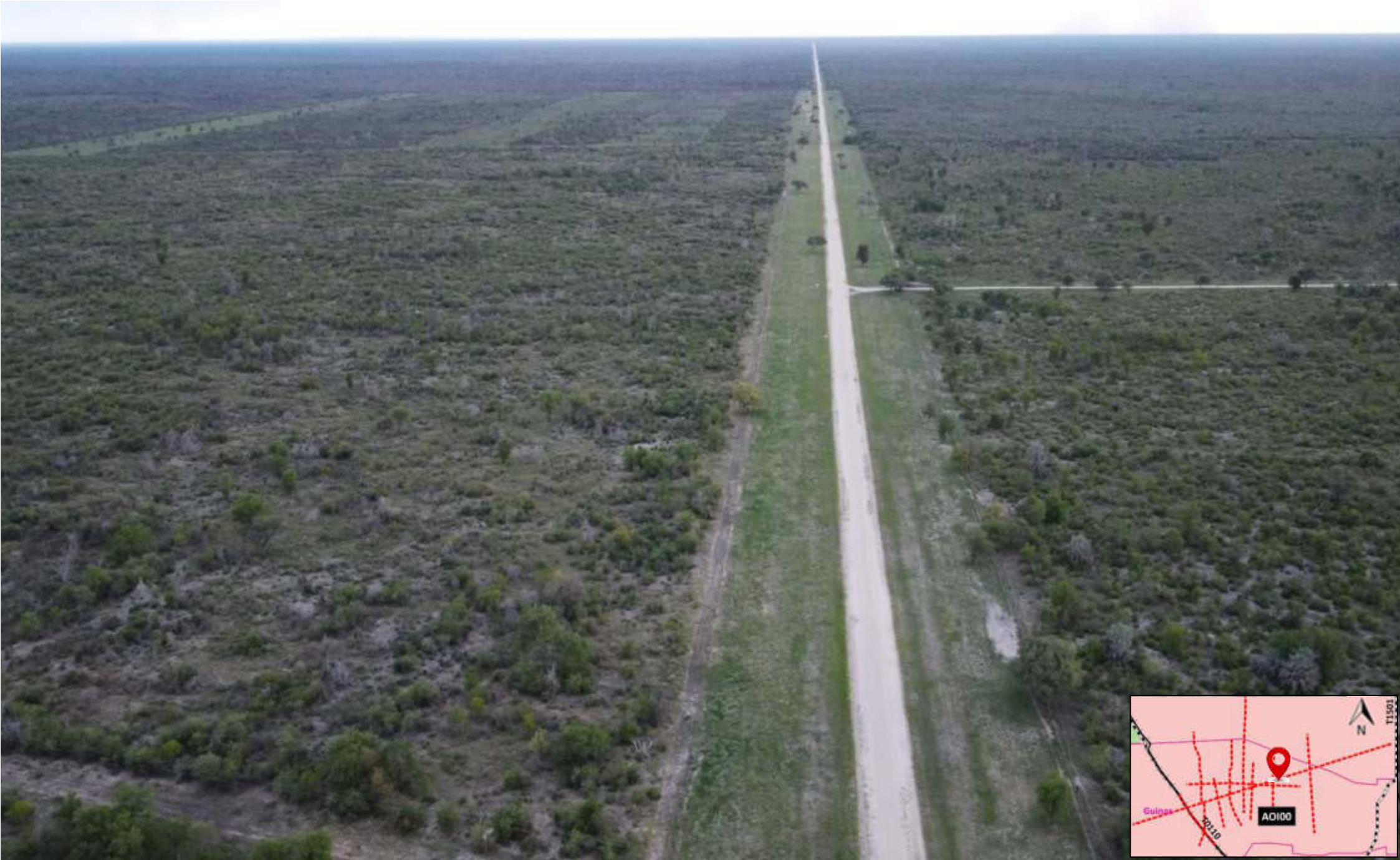
Plate 1.36: Southern section of Line 14, running along existing road D3007 to Tsumeb, drone image view to the south taken at the junction of the D3001 road linking Oshivelo to Tsintsabis and the D3007.
