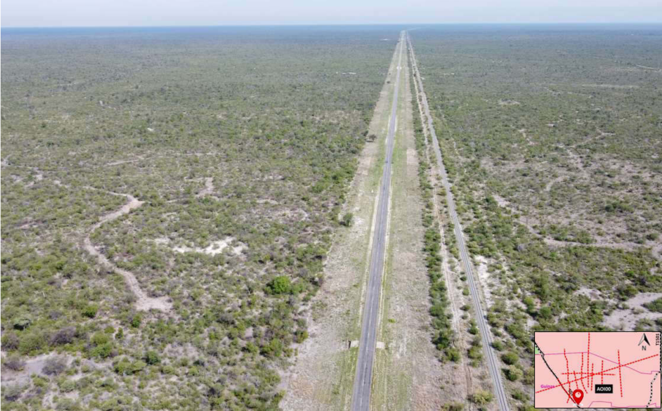
Plate 1.31: Central section of Line 11, running along the B1 Road from Tsumeb to Oshivelo, drone image view to the north taken at the junction of Line 11 and Line 10.
