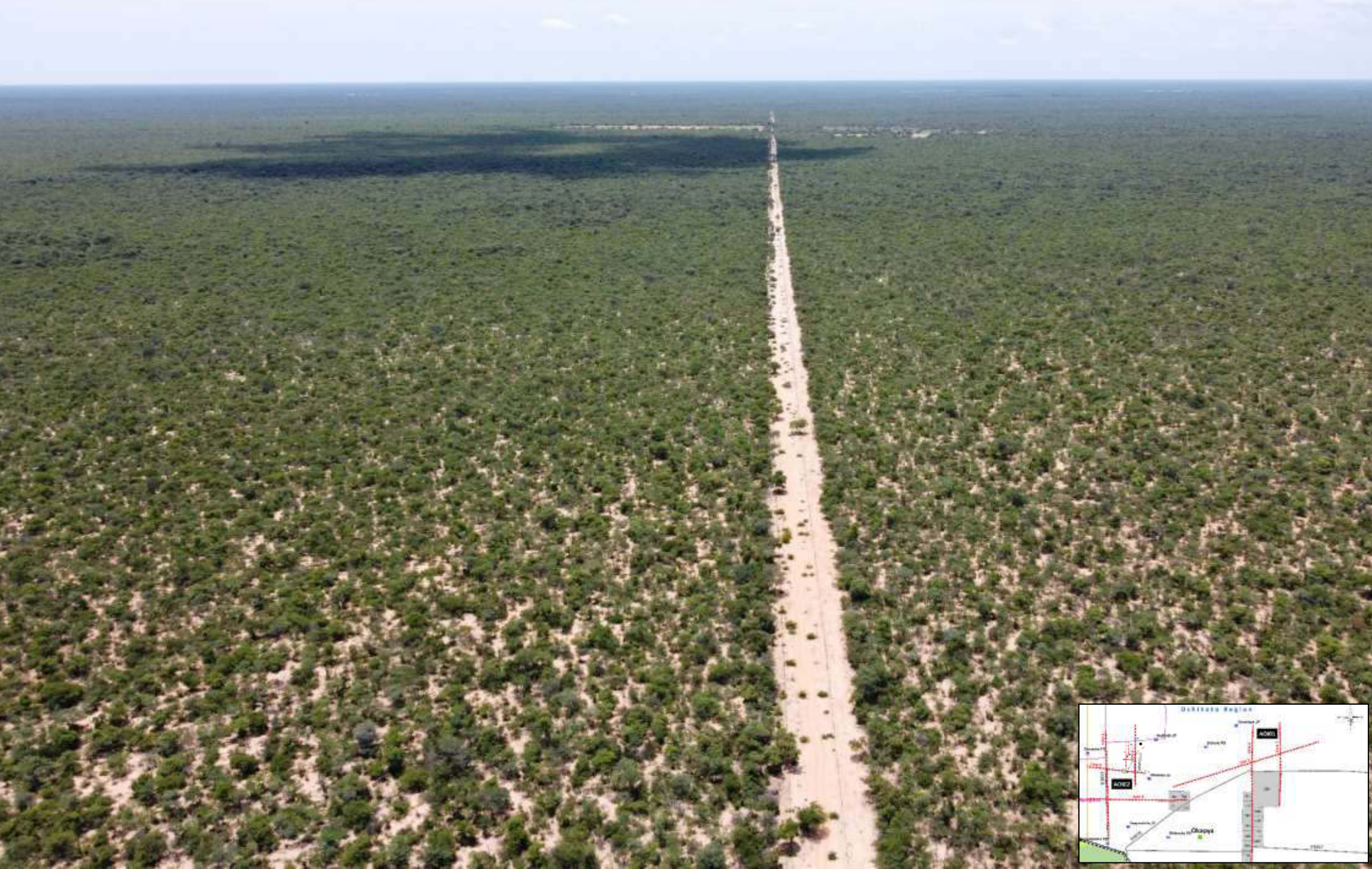
Plate 1.4: Southern part of Line 2 along existing track, drone image view to the north at the junction with the eastern section of Line 3. MEL 2D Seismic Survey Operations - 14 - EMP Report for PEL 93-APR 2022
