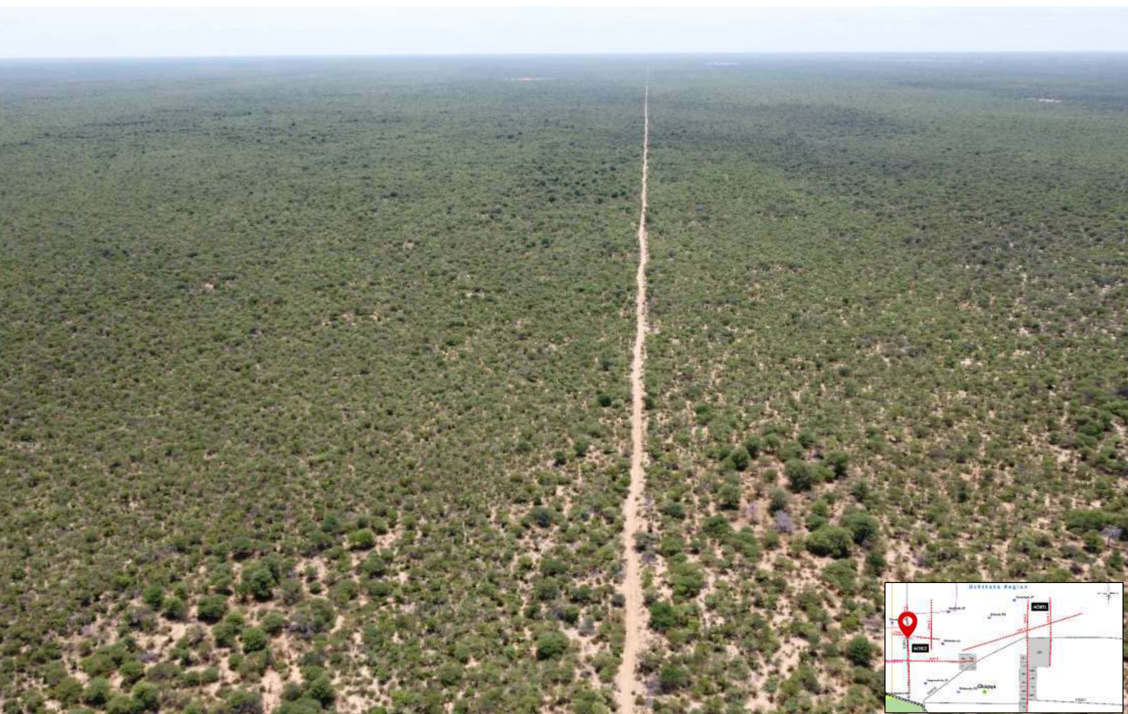
Plate 1.6: Western part of Line 3 along existing track, drone image view to the east at the junction with the northern section of Line 1.
