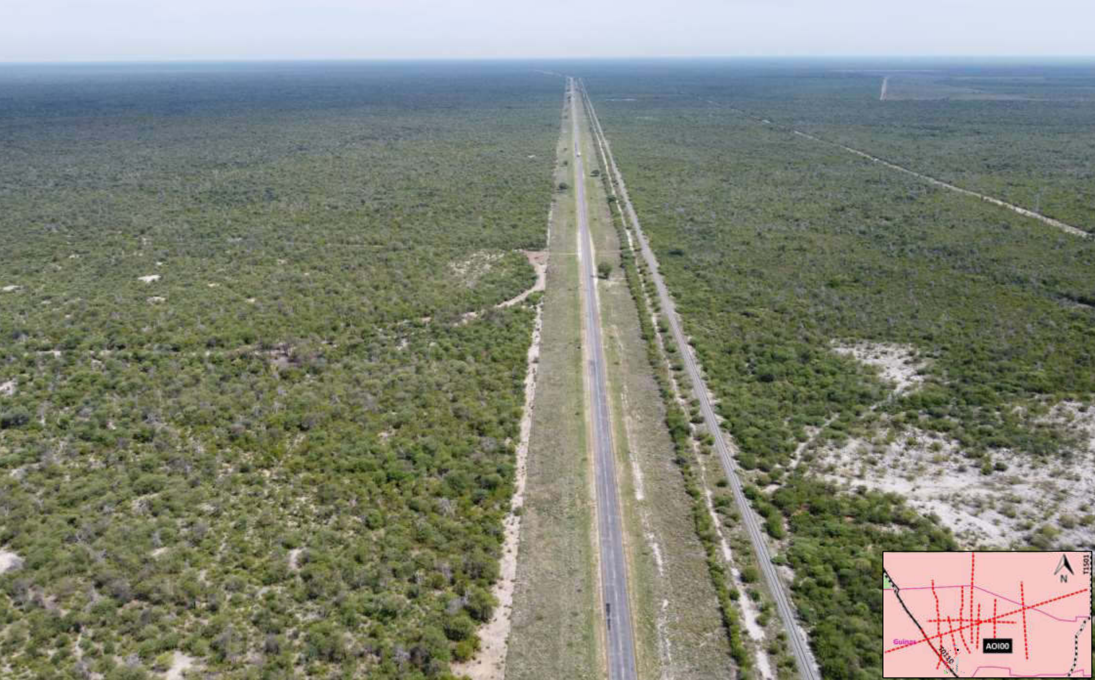
Plate 1.32: Northern section of Line 11, running along the B1 Road from Tsumeb to Oshivelo, drone image view to the north taken at the junction between Line 11 and 8.
