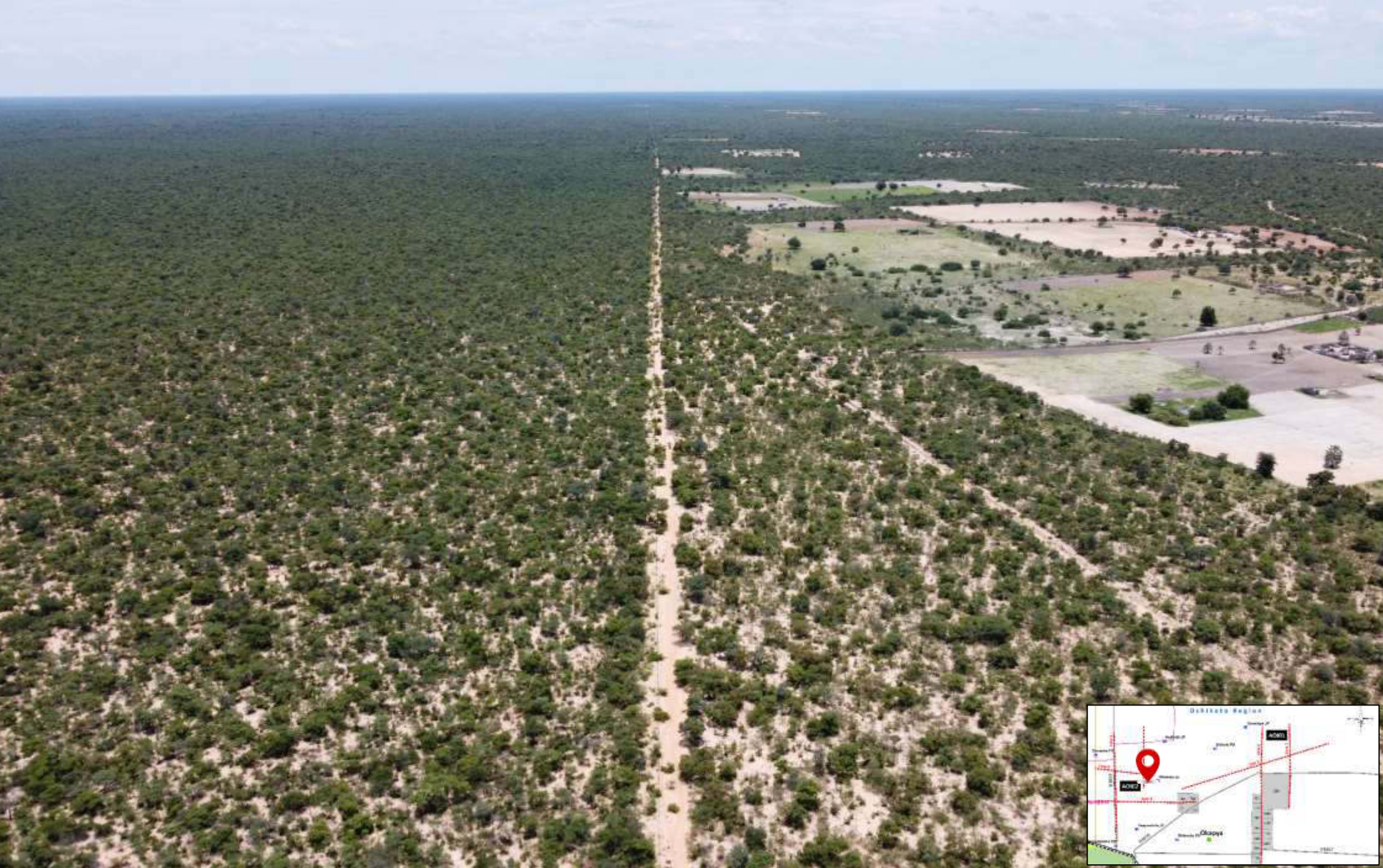
Plate 1.7: Southern part of Line 3 along existing track, drone image view to the east at the junction with the southern section of Line 2.
