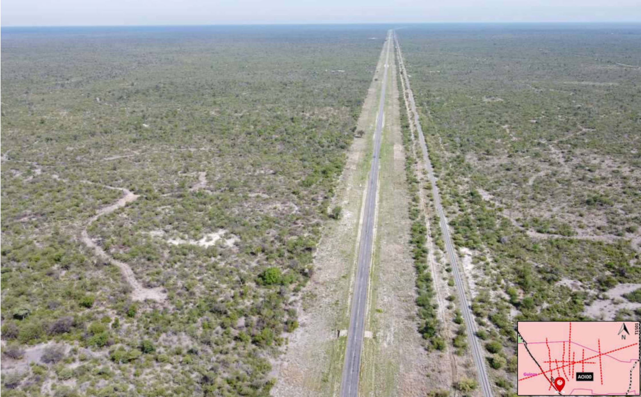
Plate 1.31: Central section of Line 11, running along the B1 Road from Tsumeb to Oshivelo, drone image view to the north taken at the junction of Line 11 and Line 10.
