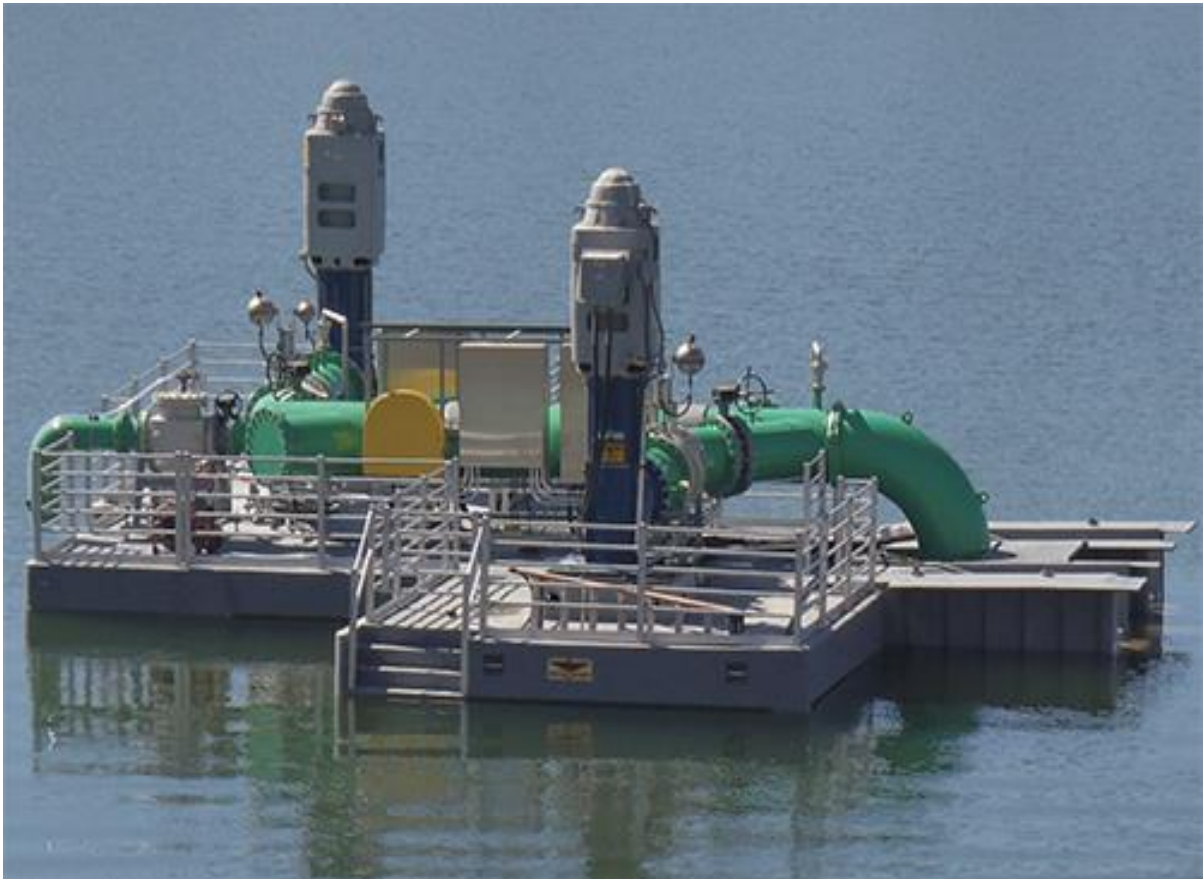
Figure 5 : Example of a submissible water abstraction from the river.
