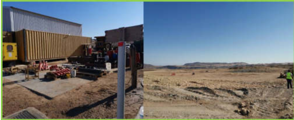
Figure 23: Before and after pictures of infrastructure removed at Obib
