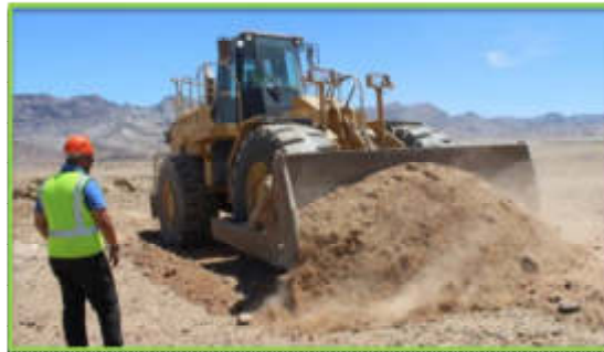
Figure 22: Topsoil harvesting at Obib
