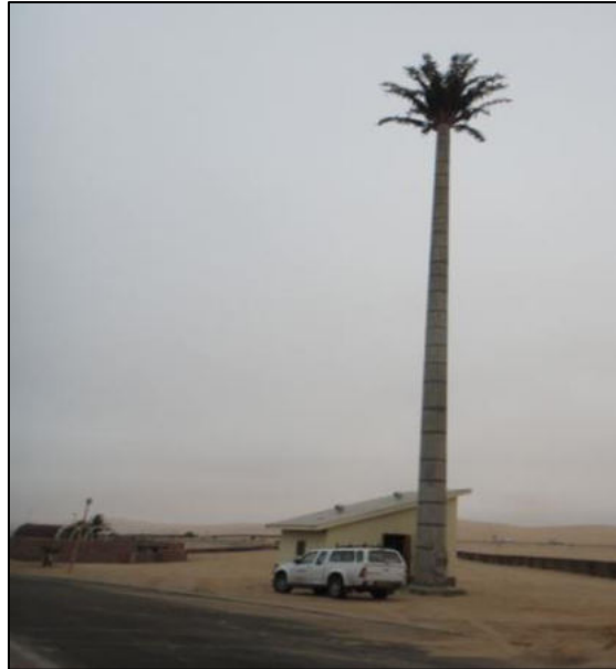
Figure 2-1: Example of the proposed tower ( https://www.powercom.na/index.php/portfolio-details/item/5-palmtree )
