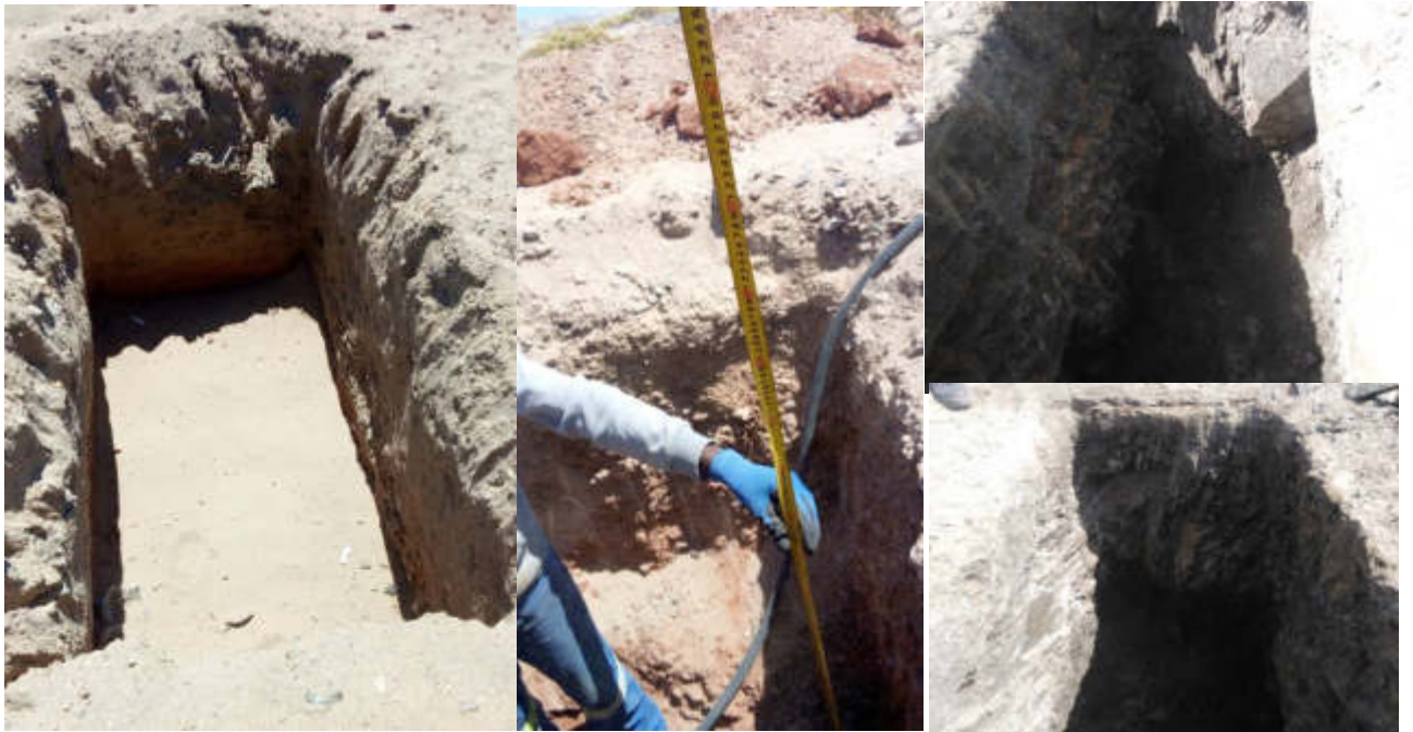
Figure 9: Pictures of trial pits
