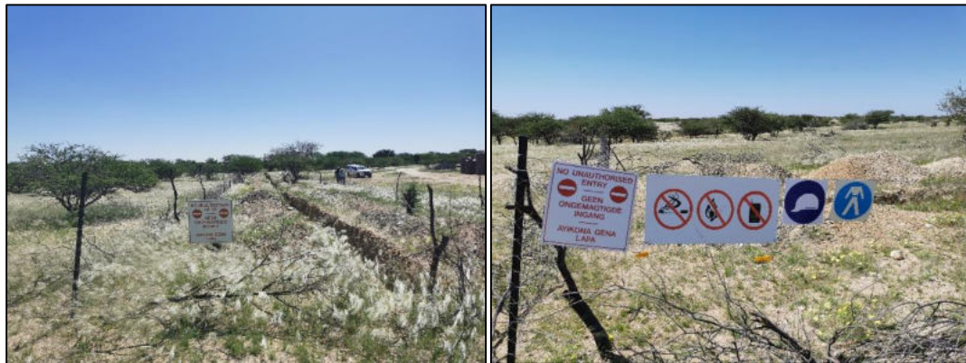
Figure 2-5: Fenced off exploration trenches awaiting backfilling upon completion of sampling (photos recently taken by Author at an active EPL in the Erongo Region (exploration auditing in 2022))
