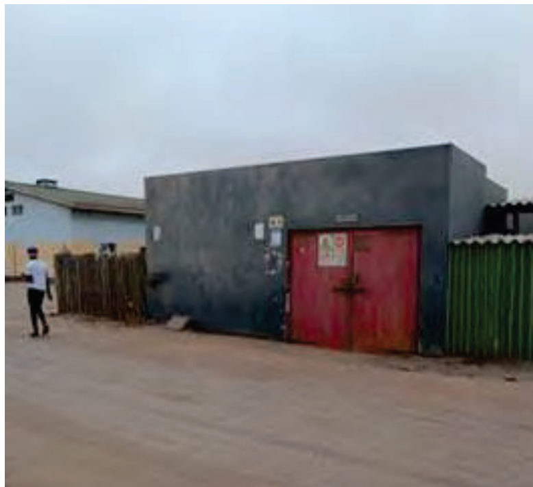
Picture indicates the Electrical Substation of Erf 1803, Mondesa, Swakopmund
