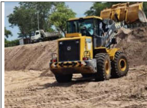
Sand mining machinery excavations and loading)
