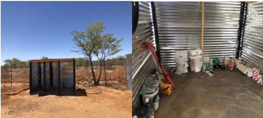
Fig2. Site toilets and materials awaiting tank from supplier.
