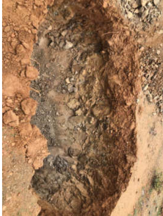
Fig2. Septic tank installation pit excavated poses a safety hazard to equipment and employees on site, a barricade tape has been recommended for installation ASAP until the tank is delivered for installation. Employees and the Site Agent have been advised to exercise extreme caution to ensure that no injuries and or fatalities may be experienced as a result of the pit.
