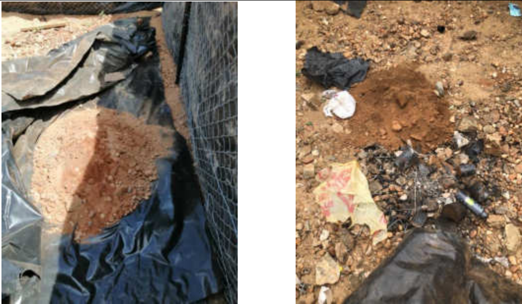
Fig3. Left: Current storage of contaminated sand from equipment oil leaks and refueling of equipment and vehicles. Right: Observed poor storage of contaminated sand because of unavailability of appropriate bins/containers.
