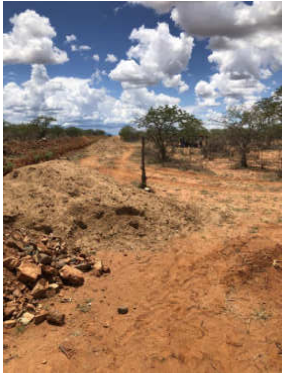
Fig2. Access road opening to the pipeline right of way to enable sand delivery for backfilling. Extreme caution has been emphasized in access road establishment, through using the least vegetated path and minimizing access road openings by making maximum use of each opened site.
