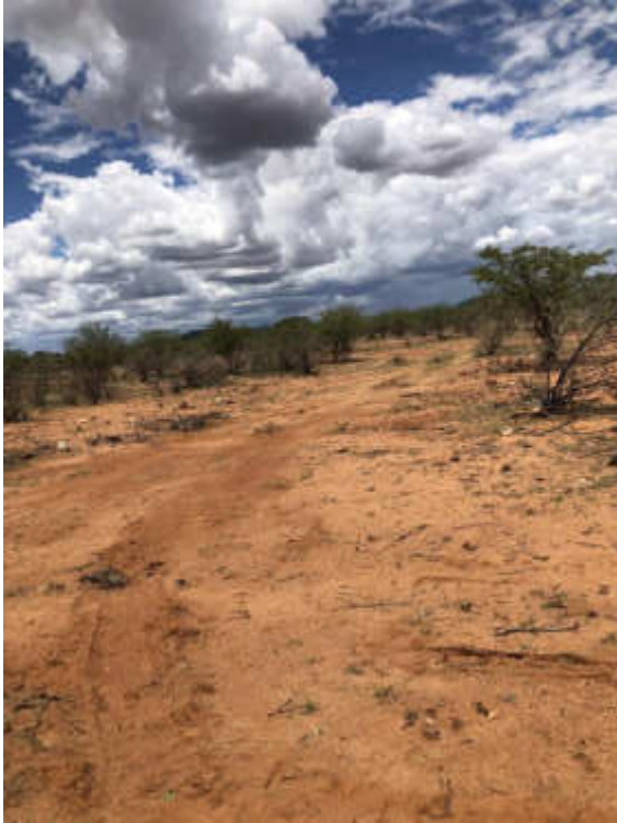
Fig2. Access road opening to the pipeline right of way to enable sand delivery for backfilling. Extreme caution has been emphasized in access road establishment, through using the least vegetated path and minimizing access road openings by making maximum use of each opened site.
