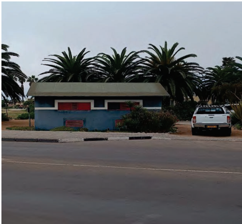
Picture indicates the Electrical Substation of Erf 92, Vineta, Swakopmund
