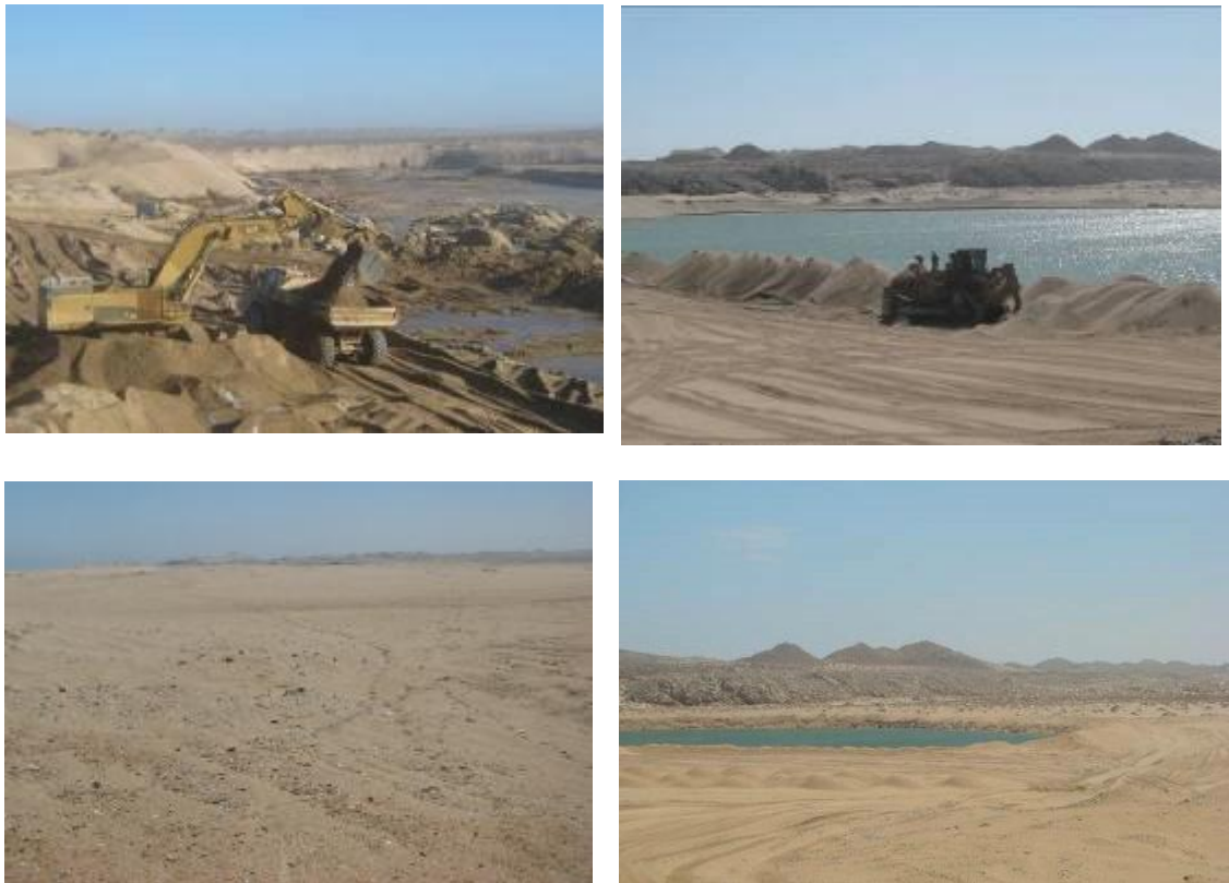
Figure 15: Large volumes of sand had to be moved to backfill the mine voids (top). Completely backfilled pond (bottom left) and remaining pond (bottom right) (Photos: Julien Cloete, Namdeb).
