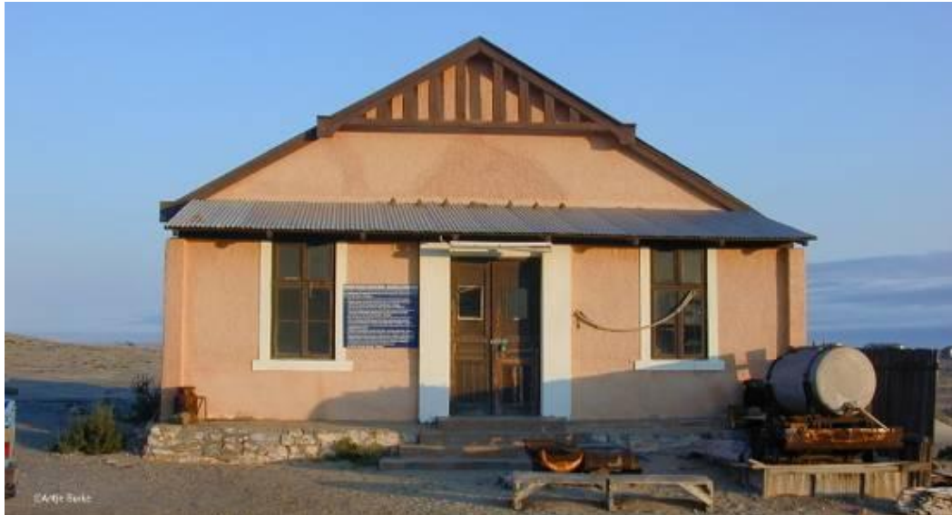
Figure 2: The former hospital at the historic Bogenfels village (the “Pink House”) has been maintained by Namdeb (Photo: Antje Bourke)
