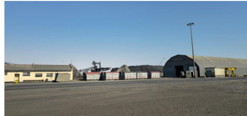
Photo 2: Coal stockpile at the Grindrod Walvis Bay Bulk Terminals located directly opposite the proposed LMTF
