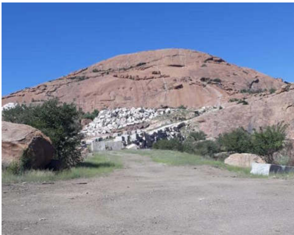
Figure 16: Cement stabilized access road onsite leading to the quarry
