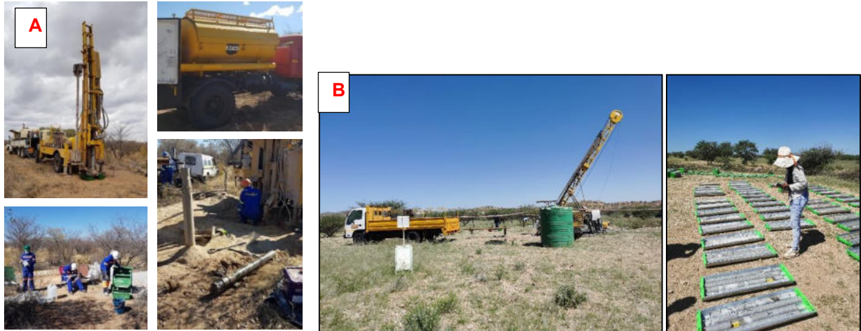
Figure 2-1: A-typical drill rig on an EPL (Resilient Environmental Solutions, 2019), B- drill rig on active EPL site visited by the Author in Erongo Region (photo by Author, 2022)
