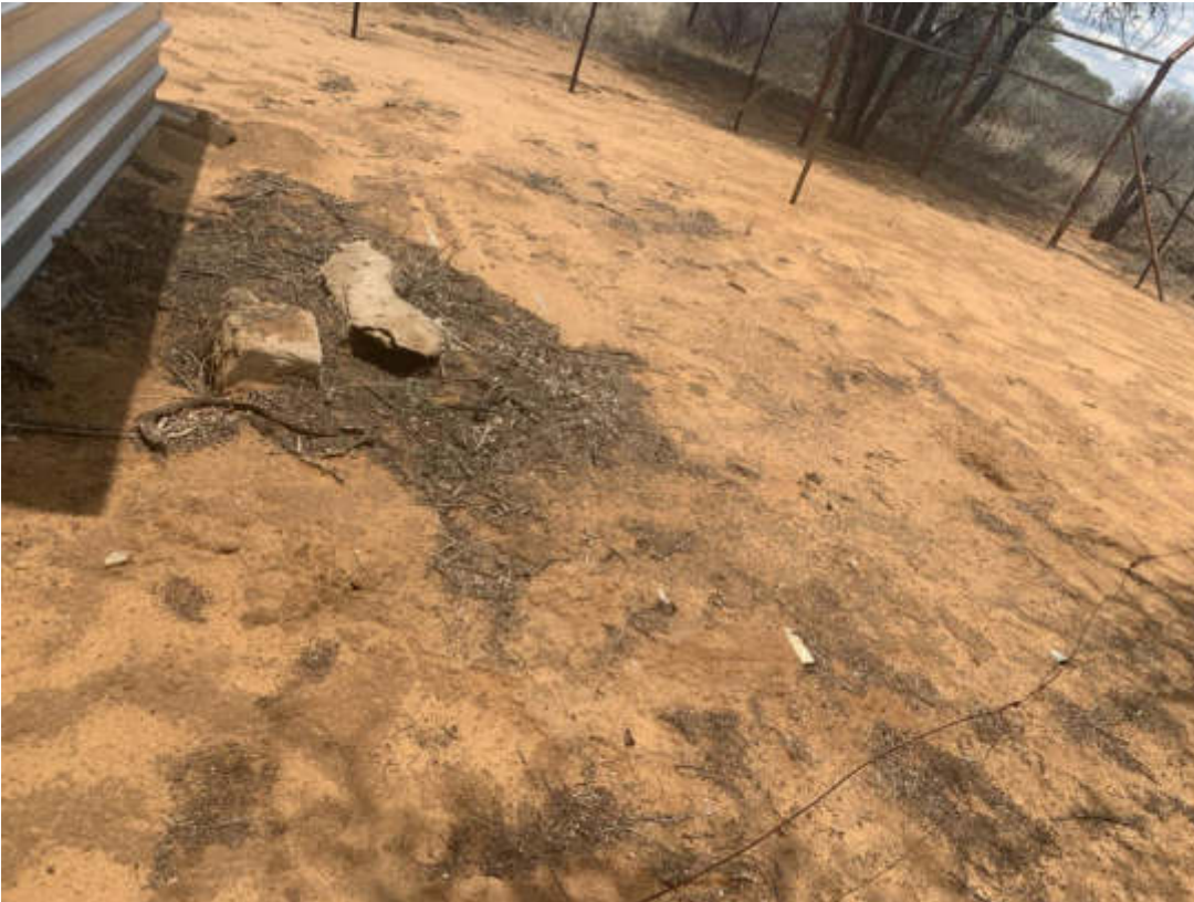
Figure 3 - Unlined effluent waste collection hole
