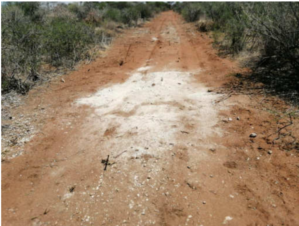
Figure 4 - The sites were rehabilitated by pouring the rock chips back into the hole, closing the hole and a peg (insert) is placed on the drill hole for future identification.
