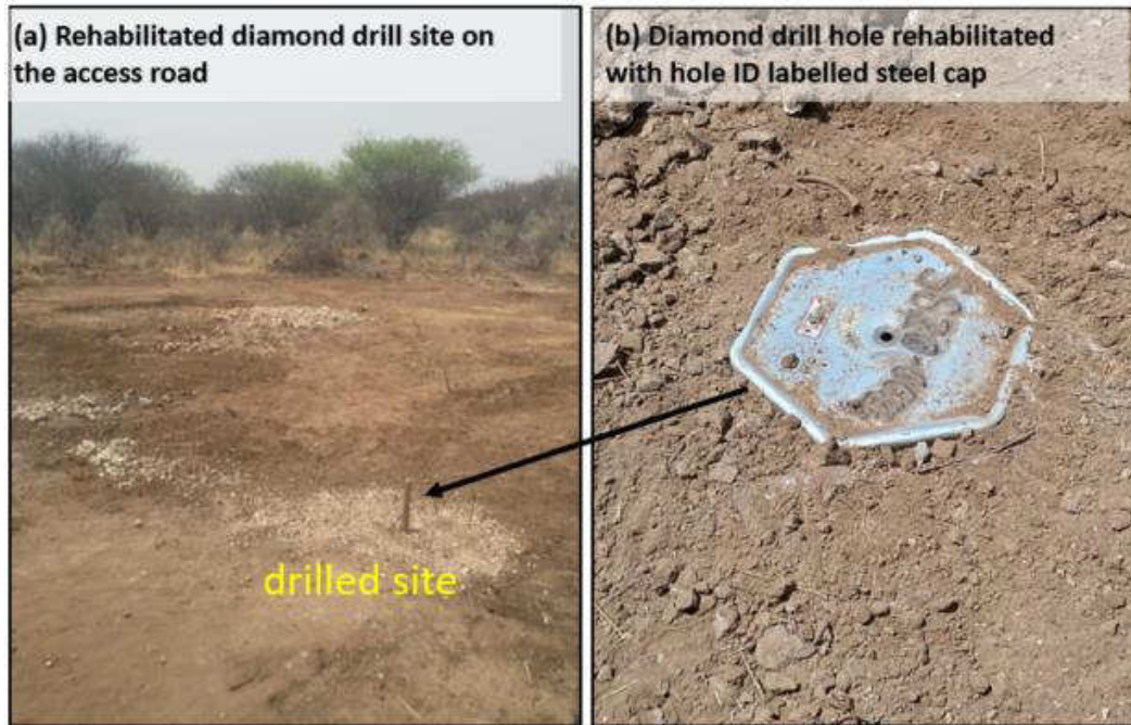
Figure 5 - Plates 3 (a) Diamond drill site after rehabilitation and (b): Diamond drill hole rehabilitated and covered with steel cap.
