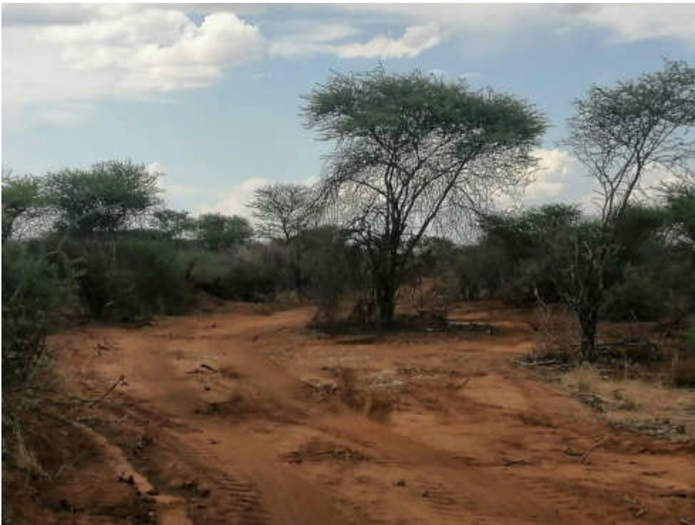
Figure 2 - Lines were cleared with a front-end loader to access the drill sites, only invasive bushes were cleared, large trees were not
