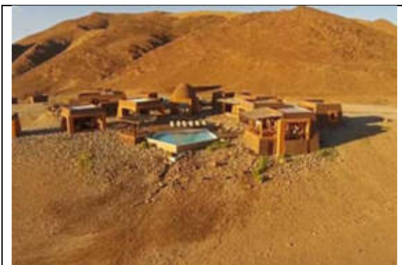
Photo 1 Lodge main complex area
