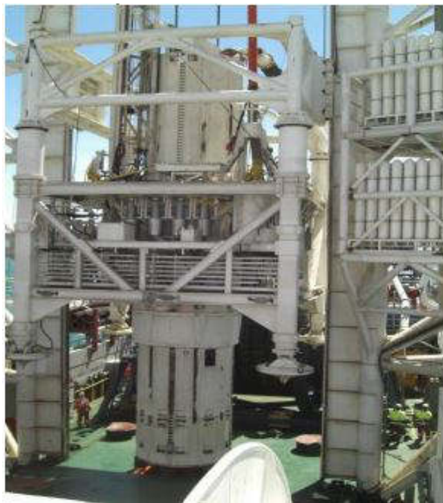
Figure 4: The 2.5m diameter drill bit within the drill frame structure.
