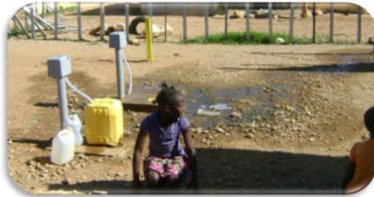
Picture 4. The pre-paid water stand pipe. Note the height of standpipes and water collecting around the stand pipes.
