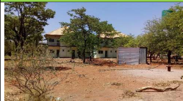
Figure 4: Borehole Drilled on the Property
