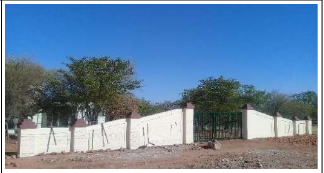
Figure 9: Main Entrance to the Lodge
