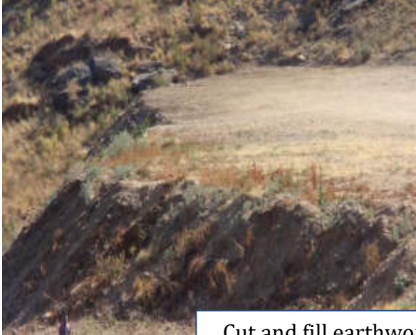
Cut and fill earthworks; and schistose bedrock
