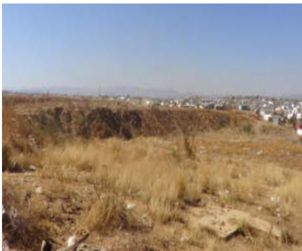
Cut and fill earthworks for landfill purposes
