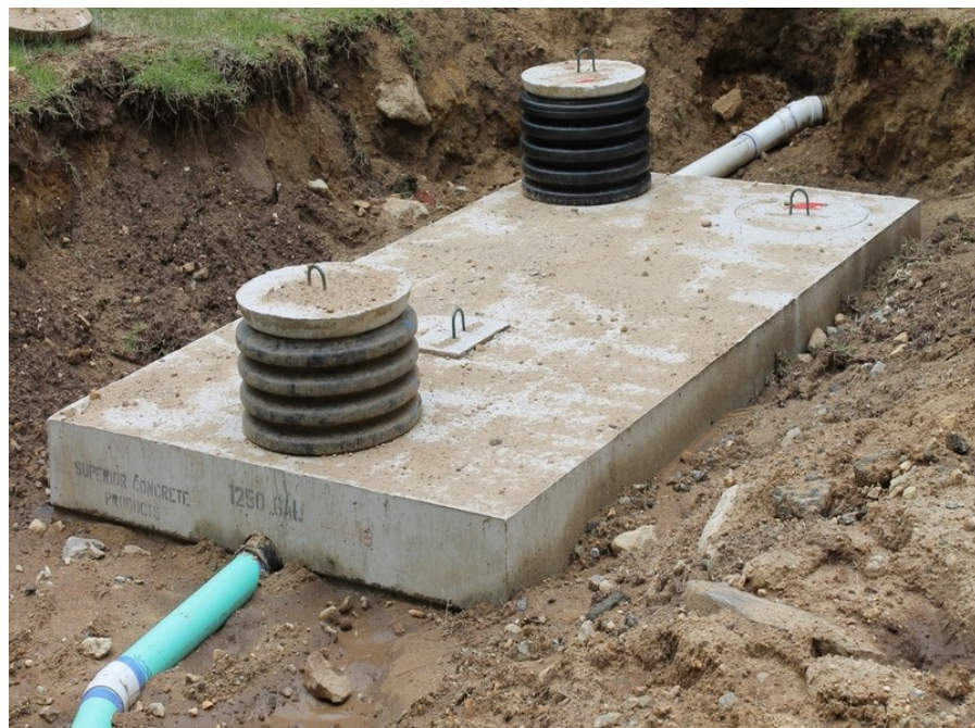
(x1) 100 000 Litre septic tank to be installed
