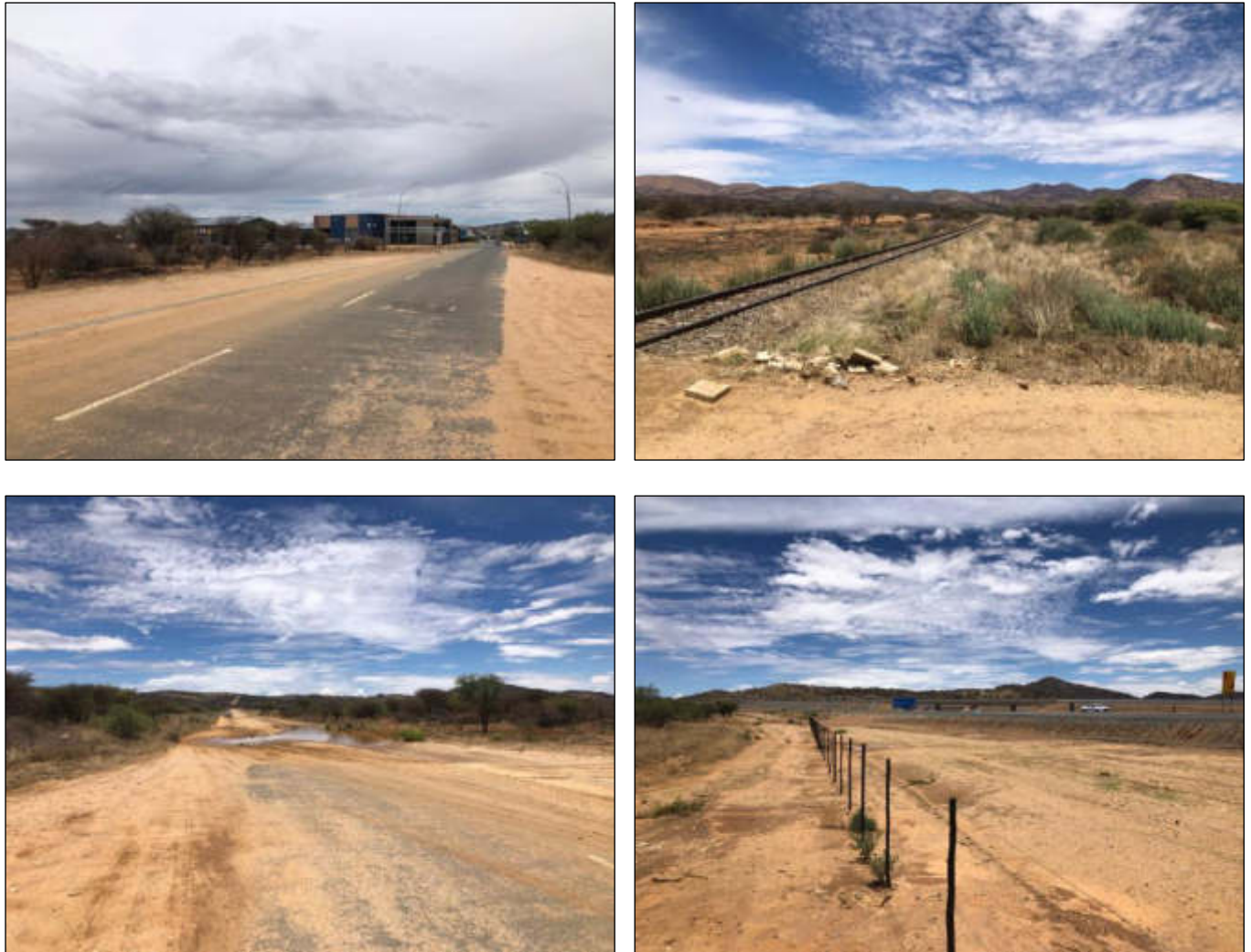
Figure 6: Project area road infrastructure
