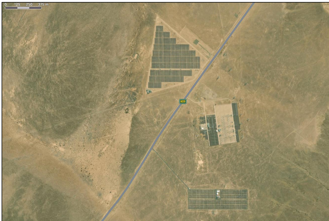
Figure 7: Photo showing existing solar plants and transmitter station
